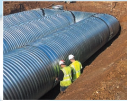
STORMWATER ATTENUATION TANK MANUFACTURED FROM HELIBORE PIPE
