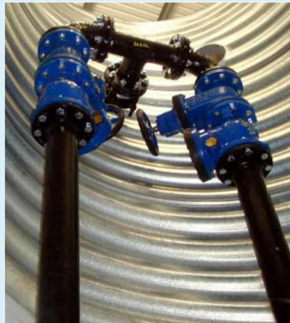
On applications where the pumped effluent contains a foul content, then the pumps can be installed as an integral part of the retention tank (having a Trenchcoat internal lining) or as a stand alone GRP package pumping station.
